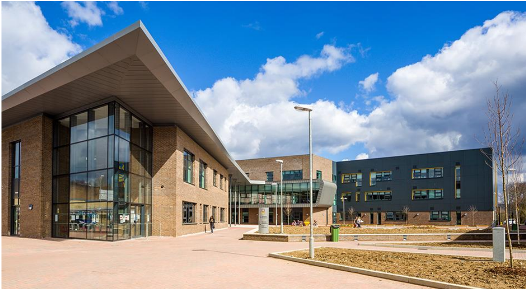
Figure 4 – Morriston Comprehensive (BREEAM Excellent) 2
